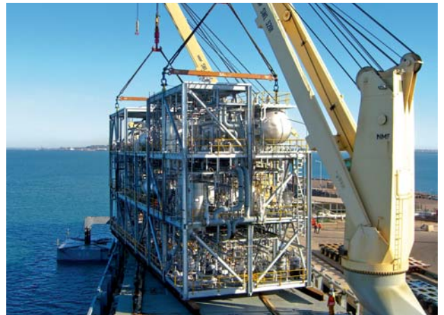
Transportation of pre-installed Biodiesel plant, Australia Capacity: 100,000 t/y
