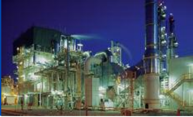
Petronas Malaysia Syngas Complex Kuantan, Malaysia
