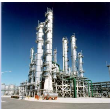
Phenole Plant, Mobile, USA
